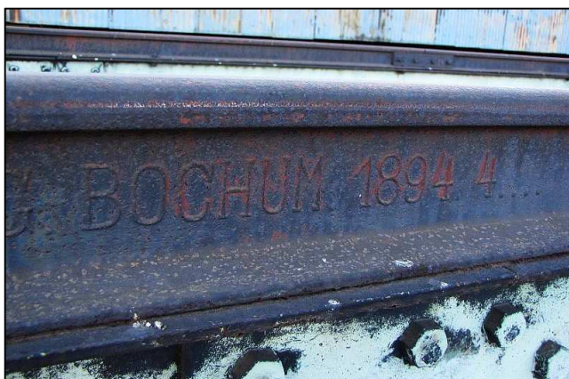
P23 - Possibly one of the oldest items we have on shed. The gantry crane's rails were rolled out in April 1894. I wonder in which main line they were originally used before they were removed and repurposed? Were they in a siding or secondary line before being used on the gantry crane?
