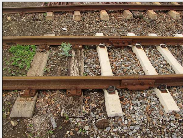
P26 – Transnet have been replacing the sleepers for the outer passing track, which is now being used as a passing loop. This station has FOUR types of sleepers; wood, iron, std. concrete and wide-section concrete. Note the bad hump over the cattle grid – the center track is not in use.
