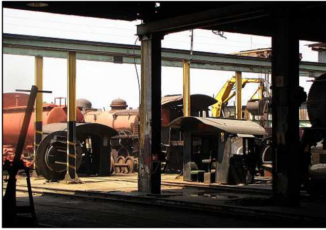
P103 - A weak point in the 15M shed operation is the lack of storage space as it was never intended to have several long term projects in storage at once and with big components all within necessary reach of the gantry crane. The 15M yard can get a bit cluttered sometimes.
