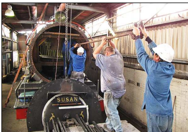
P101 - Teamwork – today it takes four fellows to slide replacement superheaters element into the 12AR's boiler flues, as there was nothing available for them to brace themselves against. The two steam-heads in the foreground are standing on the works flat wagon.
