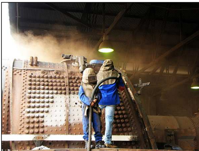
P137 - Locomotive work can often be dirty and dusty...
