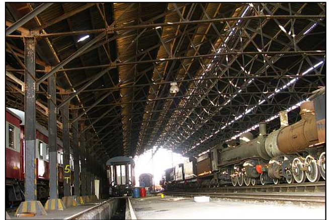
P034 - The great double barn of the old Running Shed was leased and preserved by Reefsteamers at a later stage. It is now used as our carriage and equipment storage shed. We also use it for long term storage of coaches and locomotives waiting for restoration.
