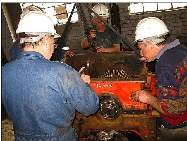
P065 - By 2013, the Shunter's gearbox, diesel engine, jackshaft and couplings rods has all been removed and overhauled. For the gearbox and drive line work, it was definitely an as-you-go type of job as we had neither drawings or documents to work with.
