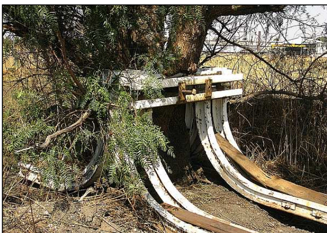
P017 - The network of tracks stand silent and begin to succumb under the relentless hand of nature. Here, a tree is actually engulfing and lifting a long-disused buffer stop at the end of an abandoned storage track.
