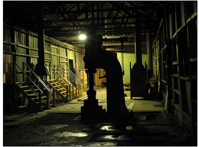
P074 - The old steam hammer in the forge house is still intact and could be restored. We have left it alone as an iron monument as to what once happened here. This open area might become a social or dining area for the future Museum with the hammer and forges as décor items.
