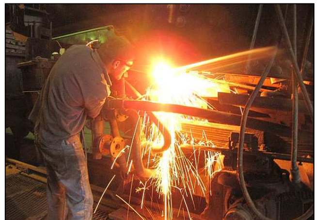
P078 - Anvils and forges aside, our guys do SO love playing with fire! The acetylene torch often comes into play for cutting away rusted fittings, bolts and rivets. Here, a rusted bracket is being removed from the firebox foundation ring for our Class 15F 2914 firebox repair project.
