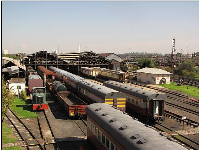
P037 - The central loco staging yard survived intact, although an assortment of coaches, goods wagons and little diesel 'critters' now occupy the rails where the steam locomotives once roamed. This scene was captured from the steps that run up the side of the water tower. (Pic 031)
