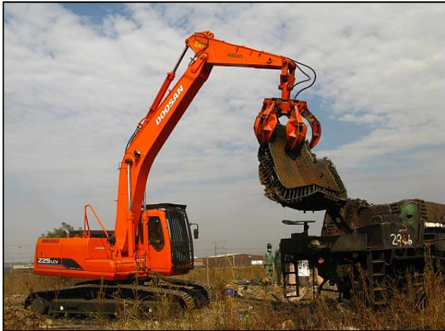
P013 - The entire top of this locomotive's firebox has been cut away. It would be cut down to several; smaller sections on the ground. One gruesomely fascinating aspect of watching a locomotive being scrapped are the real life cross-sectional views which can be quite educational.
