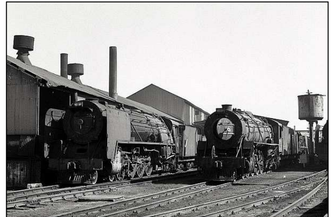
P004 - The locomotives were serviced, coaled, washed out and rostered here. Pictured is the boiler washout area. The locomotive boilers were washed out roughly once a week, the necessary steam and hot water being generated in a pair of locomotive boilers that were mounted within the shed on the left. (That boiler shed no longer exists today.)
