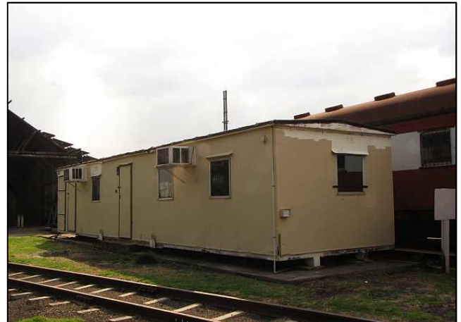
P040 - Seen in the process of being painted, this is the combination Shedman's Office and a library/archives room. The track just behind is the coach repair/storage track. This building might soon be converted to house delicate indoor exhibits for the Steam Museum.
