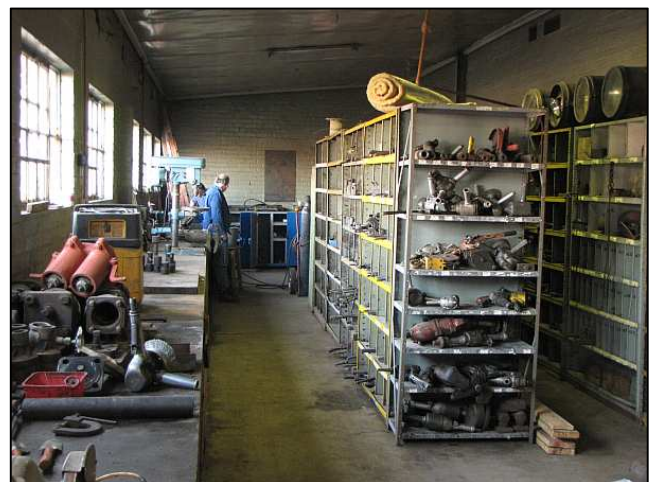
P084 - The old fitter's shop has been put back into service to get the tools, small supplies, fasteners and workbenches all back into one location. It still needs a lot of work on the lights and the leaking roof.
