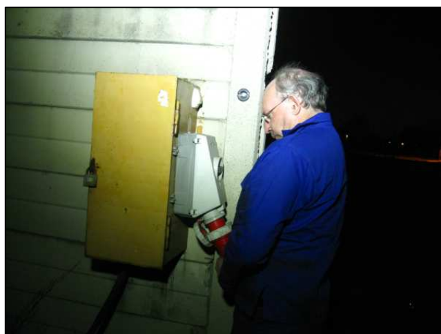
P38 - Aidan battles to connect the 3-phase 'extension cord' as the rubber weather seals go stiff in the cold weather. The grab's heavy electrical cord is now a plug-in, as it has been stolen several times. We lock it away between uses.
