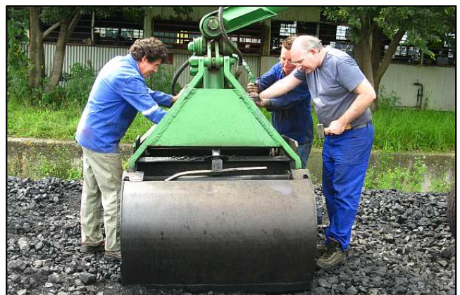
P12 - After uncoupling, the actuator's innards were removed without removing the cylinder, by using the hydraulic pump to force it out. It was quite awkward getting everything back in again through the canted cylinder and then trying to get the worn cover bolts to line up through the scraper, the tightly fitting end cap and the actuator body – and working upside down as well. They managed it!
