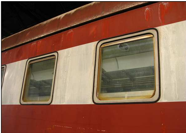
P15 - Here's a problem the coach boys found! Dusty's windows have a fibreglass cowling as an insert (see the extra rubbers?) and they do not match those of our other coaches. The window glasses are a lot harder to remove.
