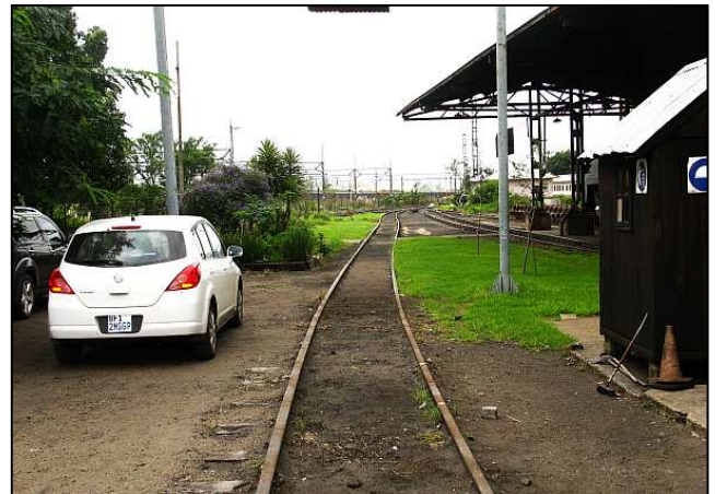
P10 - This is where the axles came from. This track is to be lifted back to the garden and buffer wedges welded on the ends. This means that a bakkie or a truck can now drive along over one rail of that track and stop opposite the clubhouse from unloading for special functions.
