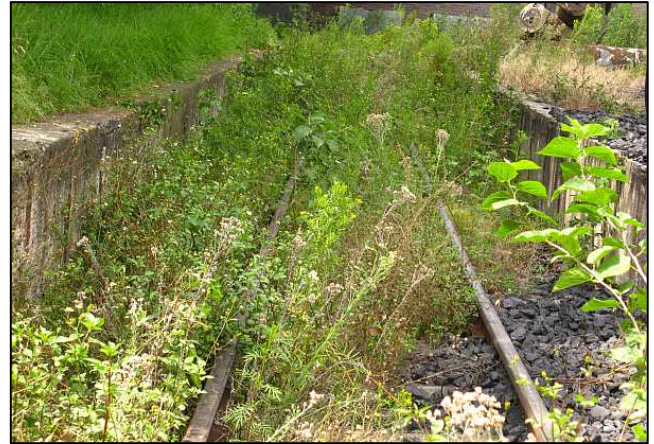
P08 - With the depot being closed for two months over a hot, wet summer because of permit issues, the weeds have taken over the entire site and we are still battling against their head start. This is the overgrown coaling dock.
