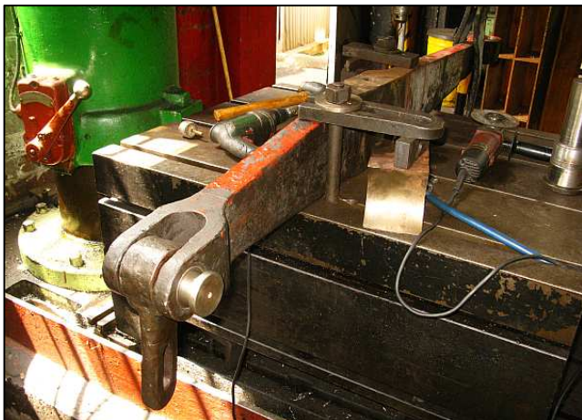
P07 - It took some ingenuity to get this awkwardly-shaped work piece clamped to the drill table! All three of the holes were cleaned out. The spring shackle end received two new bronze bearings – but with a deliberately loose fit.
