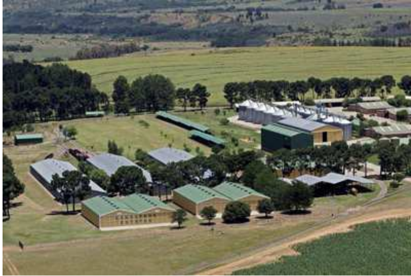
Photo 2 caption: This is an excellent photo showing the three main Heritage buildings at Sandstone. The one on the left contains traction engines and classic agricultural machinery. The middle one is the Running shed, and the one to the right contains our coaches and valuable items of rolling stock. Unrestored locomotives which were previously restored here have already been moved to the big new ex Ficksburg shed.
