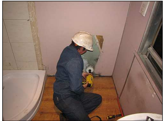
C26 – Alan has a go through that wall with his 110mm diameter hole saw. Unfortunately the teeth no longer have any set and all the saw was achieving was scorching a groove into the plywood. And that stuff REEKS when it gets all hot and smoky!
