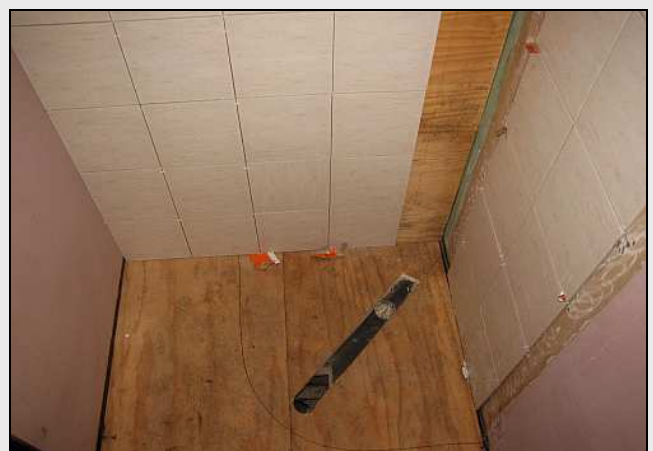
C12 – A view looking down into the shower-to-be. The tile cutter purchased for the job wasn't able to handle the floor tiles. That dead space in the left corner will allow continued stand-up and 'bunk steps' access to the standard overhead storage which extends over the corridor ceiling.
