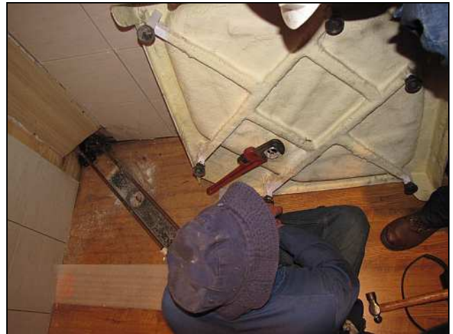
C22 - The grotty and badly siliconed Setimela-era drain fitting was replaced after the levelling operation. The fellows had to turn the body against the drain's grid to get it loose, but they managed without fracturing the shower's fibreglass pan. (Sighs of relief all round.)
