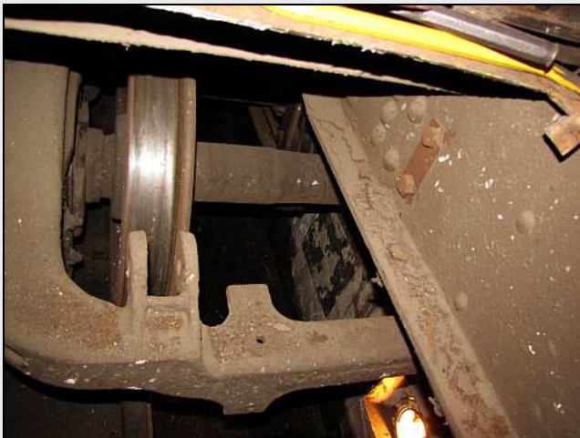
C03 – Seen through the new hole, you can see how the wheel would spray water into this area. As the vestibules are designed to be crumple zones, there is no corrugated under-frame plating here, as per the habitable spaces.
