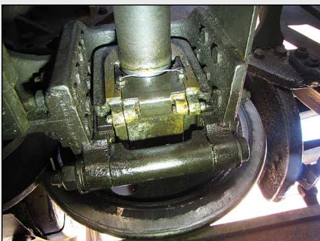
W05 – While working under all the iron, the fellows checked other bolts and safety wires as well. A good habit to have! Seen is the detail of one of the bronze front bogie bearings, with an oil box packed with oil impregnated 'socks.'
