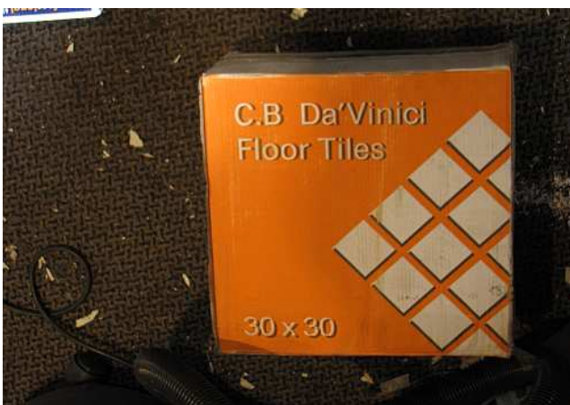
C11 – The decision was made to go for oversized floor tiles rather than normal bathroom tiles. It would reduce the number of grouting joints to be made, and the silicone would help prevent cracking. We would have still had the same number of tiles to trim, regardless of their size.
