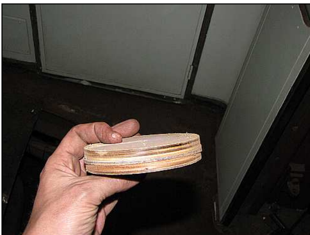
C27 – The chaps eventually cut the hole with a tungsten jigsaw blade and some swearing. In the resulting 'biscuit,' you can see the double five-ply of an UCW Coach firewall – with the fire-retarding steel plate right in the middle.
