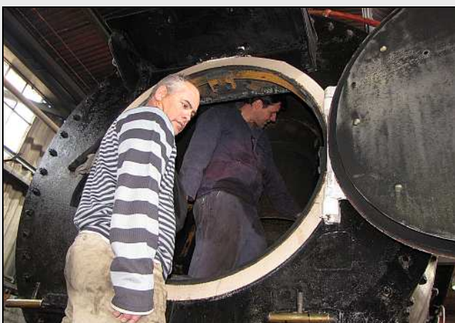
P03 – Michael (L) and Dawie (R) confirm that they are to start with opening-up the Steam Delivery Pipe Flanges for inspection of the front-end steam leaks.
