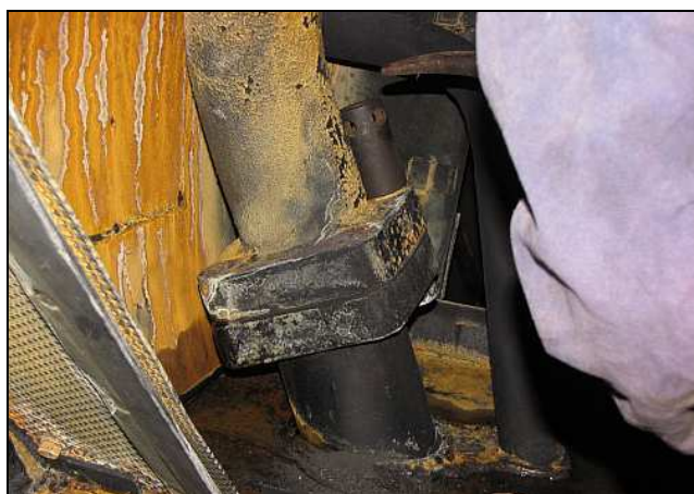
P04 – The RHS waist flange is being dismantled to inspect the blown gasket – note the thoroughly steam-cleaned smokebox barrel.
