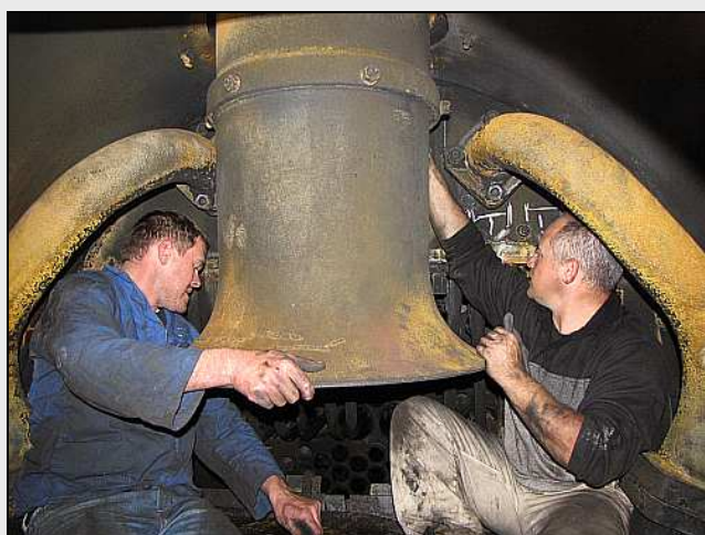
P06 – Smudge (L) and Rekots (R) start undoing the long-cooked bolts holding the petticoat into the chimney. Dawie had spanned the chimney with the shaker lever by now and was fetching a chain hoist.
