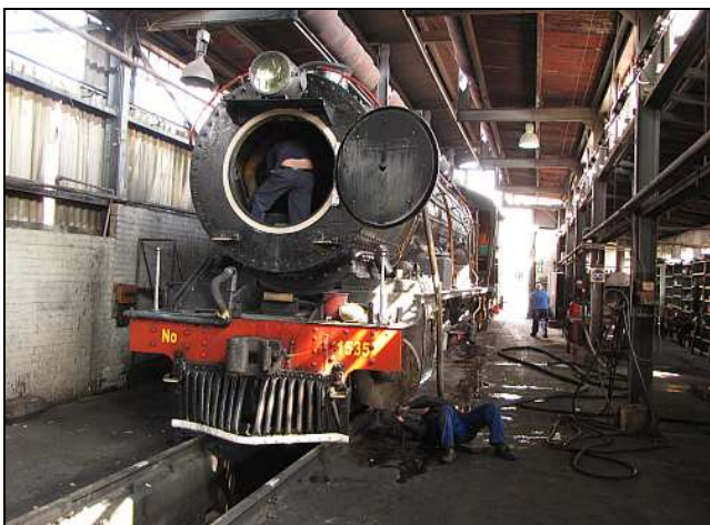
P01 – Taking a break before the busy June season, Class 12AR No.1535 ‘Susan’ is undergoing running repairs on the cylinder cocks and superheaters.
