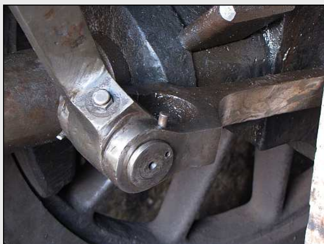
P10 – Class 15F 3046 – A clevis-type joint at the leading end of the Union Link, still clean with a new Vesconite bushing installed. (This provides the valve event cross-head lead for the Combination Lever.)
