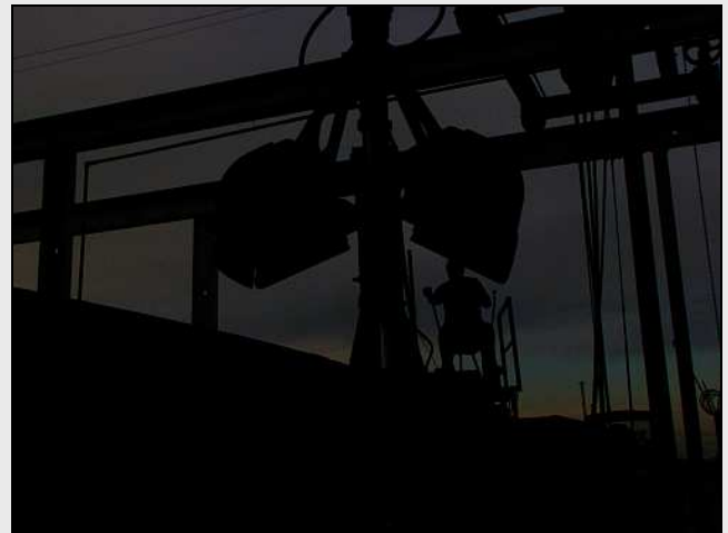
M10 – Parking the Coal Handling Wagon’s Boom away after a long day. The clamshell buckets have since been dismantled and the bent sections cut out, pressed flat in the 50 ton hydraulic press and made ready for re-welding.
