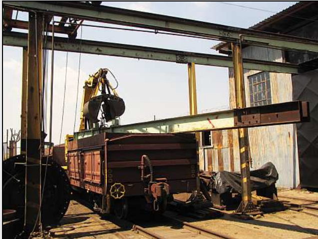
S01 – The ex-SANRASM Tube Swager was dismantled into 2 main pieces and the upper set of beams were moved on Sat, 23 March. Here, you can see the upper half waiting to be unloaded, using the Wheel Lathe's gantry crane.
