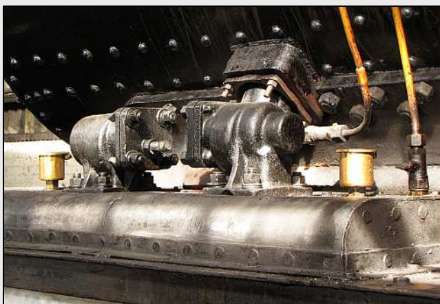
R07 – A view of Susan's recently-painted bypass valves. The steam down pipe is currently sans its cowling for quick rectification of any stuffing box or gasket issues. The horizontal sparkplug-like device is the steam oil atomizer.
