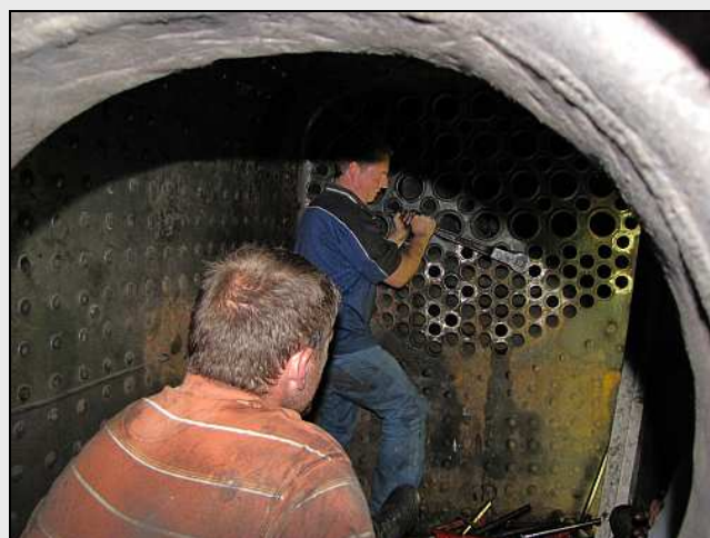
L12 – While Simon is now wrestling with another weeping tube end, Shaun has to make a call to go on or quit. Tubes cannot be just expanded indefinitely as it spreads the metal, thinning out the tube walls as well as the ferrules.
