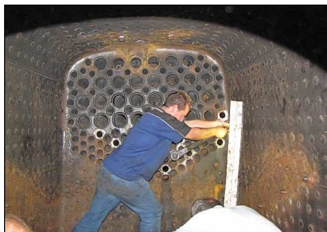
L10 – Simon gets a-going with the ratchet and driving the tube expander, with the boiler at about 1400kPa. As you can see, we slipped up a bit and had neither the firebox or tube plate cleaned properly, which was another reason why the Boiler Inspector was a tad grumpy on Wednesday.
