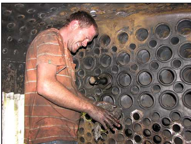
L15 – Yeah! See that happy bit-more-encouraged smiling face now! (A grumpy Smudge is not pleasant to be near and throwing soap at him doesn't keep him at bay.) However, this would be the last attempt at stopping that flue tube from weeping with the risk of over-thinning those tube walls or 'smooshing' the ferrule within the tube plate.
