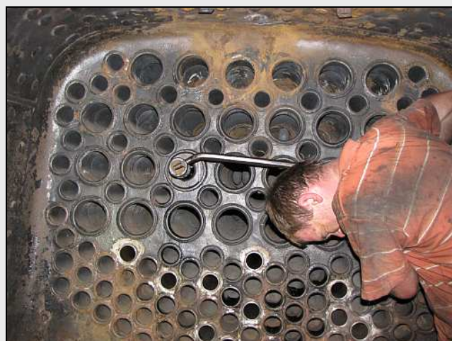
L16 – He is really putting some grunt onto this one! (Boiler is at 1600kPa.) What makes this tricky is that water gets into the doughnut-shaped cavity between the bead and the copper ferrule. When the tube is expanded, the trapped water is squeezed out under pressure. The trick is to work out if it is a squirt or a leak before over-expanding the tube.
