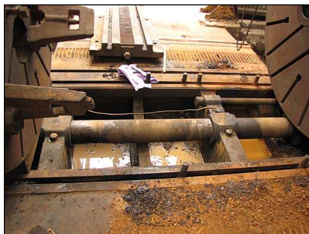
W10 – This was the state of the transfer shaft pit with the project just started. Although the lathe itself was covered in a tarp, water still got into the building through the decayed roof. Note the oil line running to the center bearing.
