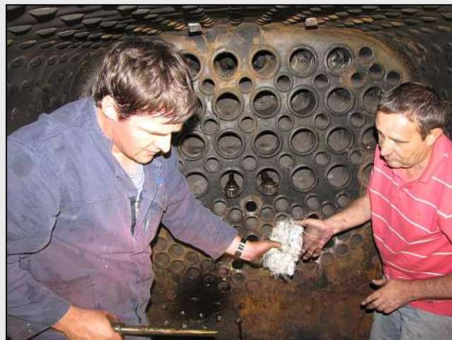
B10 – Hmmm. Hardened steel, homogenous core, 10 inches long and very inflexible. 'The wand chooses the wizard, Mr. Viljoen.' Although a bit of oil is needed to reduce binding, the debris quickly gunk-up on the oil-wetted mandrel. Jeremy passes the waste across for a quick wipe.
