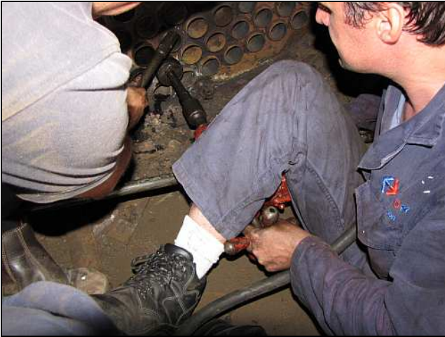
B13 – At the end of a good expansion job is the need to get the expander and mandrel out again – with the rollers squeezed in TIGHT between the tube and the mandrel. Michael gets a bit of rap action going. Note Dawie’s cute and still miraculously clean white soddies in those rugged work boots – this dude is STYLIN’ !
