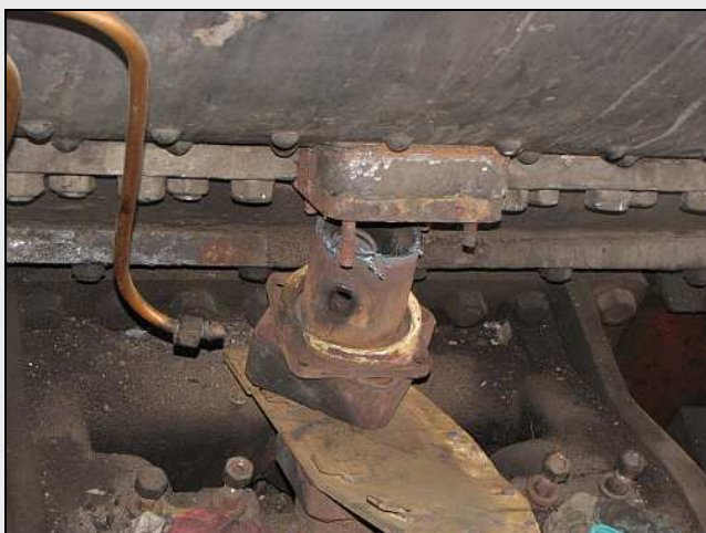
R13 – The heavy flange drops onto the baffle plate and is left to cool while the inner section of the pipe is withdrawn. The rotated square piece is the loose stuffing cover for the upper joint – sealed with graphited rope as packing. The cover is relatively lightweight, as it is 'only' a vacuum joint.
