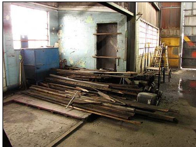
M08 – The wooden floor boards of the recently demolished tools store now hold the rotted roof rafters removed from the wheel lathe house's roof. These are in storage for use as locomotive fire kindling. And a Viking's funeral is not an inappropriate way for old SAR&H timber to be laid to rest!
