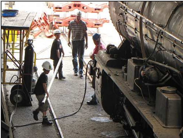
C07 – The short ‘uns get to take a new boiler tube in all by themselves this time, without Jeremy getting up to mischief at the tail end. In the background are the buckeye bogie frames for Greg McLennan’s 24 Class’s tender.
