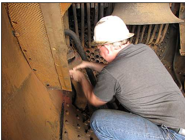
B11 – Aidan gets his 'grunt on' and wrestles with that now-warm pipe. For full access, the wing pipe from the dry side of the superheater header should have been undone first. This way was harder, but avoided breaking open an extra joint.
