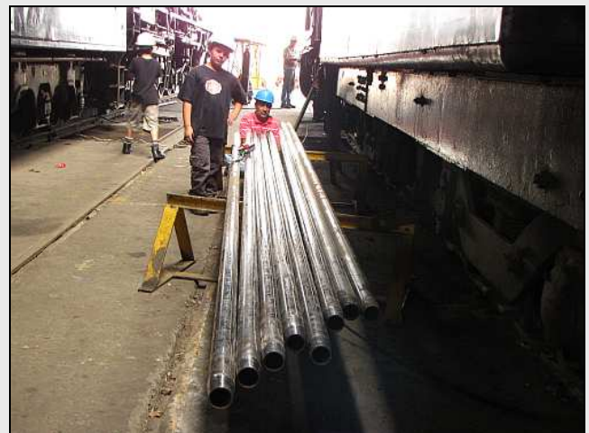
C12 – Jeremy grinds down the burrs on the insides of the newly cut tubes while Gabriel supervises. The tubes act as great sound pipes and I could hear the grinding clearly from the other end. It’s always weird to be able to clearly hear someone talking in a firebox when you’re in the smokebox.
