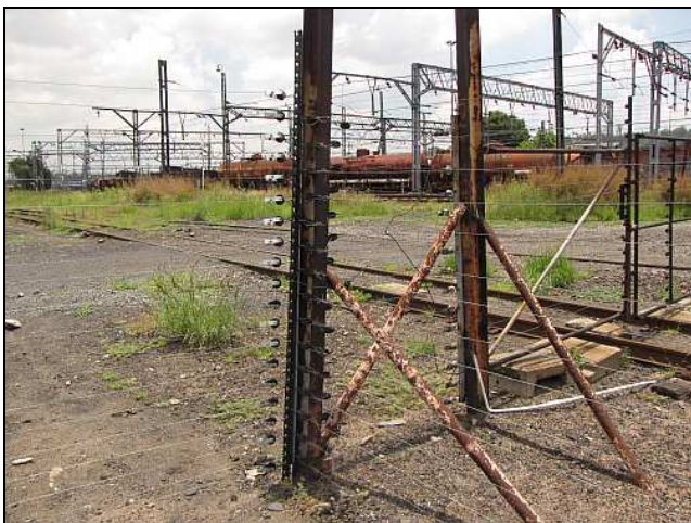
G03 – This is the complicated junction wiring between the new balloon fence (left) and the existing western yard fences. This area will later be rewired to incorporate the new gates into the western yard wiring, and to terminate the already-long balloon fence at the other corner. Thus, a fault at the complicated gate wiring won't compromise the new, longer fence protecting the Turning Balloon.
