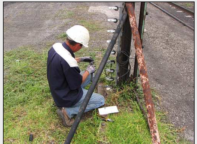
E12 – Alan gets to (gloved) grips with installing new jumpers on an existing pole at the members' driveway entrance. With the removal of the paddock fence, some of the alternating polarities of the fence strands were incorrect. Note that one of the gate braces is a boiler tube!
