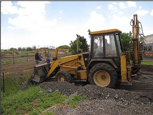
E09 – Here is the very useful TLB that we had been using on site for a few weeks. (Not for free but we did get a good deal!) The three gents are in the background, not in the bucket! The operator is pictured filling a ditch that has long been an ankle twister and a parking space waster.
