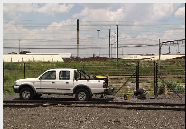
S06 – A general view of the work area. The fencing contractors didn't follow the instructions to maintain a 3m gap between the tracks and fence, so the outer road is just a bit too narrow for a full sized vehicle. But the outer path is to be used by security guards and later, a dog patrol.
