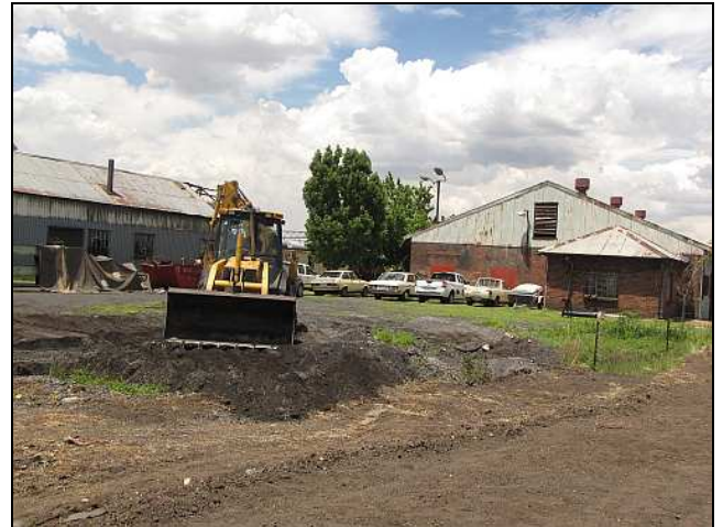
E10 – The existing car park wasn't altered much, but the collected soil and ash was being used to level the old paddock which occupied the corner. This area is currently being covered with our locomotive ash, which works well at stabilizing raw ground and as a high-traction ground cover.
