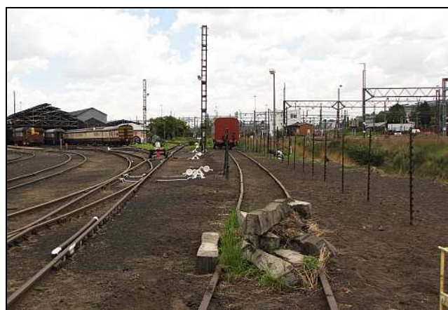
E06 – The fence poles seen on the right side originally ran up the center of the track. Being the thrifty skinks that we are, the poles and insulators are being reused but all the strand wiring is being replaced. The trackwork and surrounds were cleared and levelled a week previously via a combination of front-end loader and man power!
