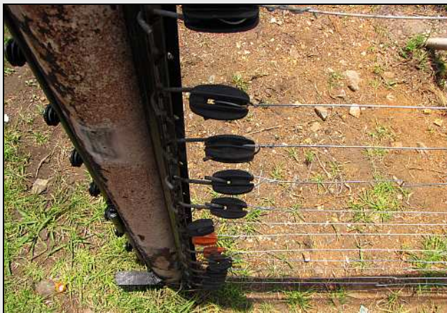
S03 – Another view of a completed stopper at the bottom of a pole full of cleats. Some of these cleats have been installed incorrectly as the hooks were too short. But they continue to do the job electrical-wise.
