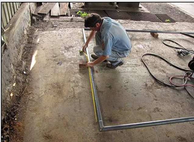
G21 – Alan Lawton marks out the spacing for the insulator bobbins, preparing for the tedious job of drilling out those poles. That is a brand new tape measure too, as the previous one died after a few days of rigorous Reefsteamers usage!
