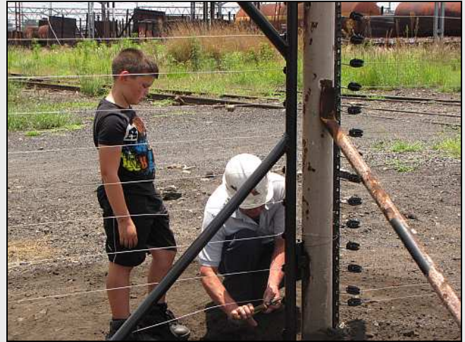
G08 – Alan takes over to put Gabriel out of his misery. Notice the little 'pip' on top of the gate hinges. That is a grease nipple which were tapped in the previous week. As the gate barrel hinges are counter-hung (So you can't just lift the gate off), the pins cannot be exposed for lubrication.
