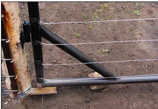
S01 – A view of a recently installed gate stopper. Its main purpose is to prevent the plastic insulator bobbins from being crushed against the pole if the gate is swung too far open outwards. The inner swing radius is inherently restricted by the diagonal braces for the gate posts.
