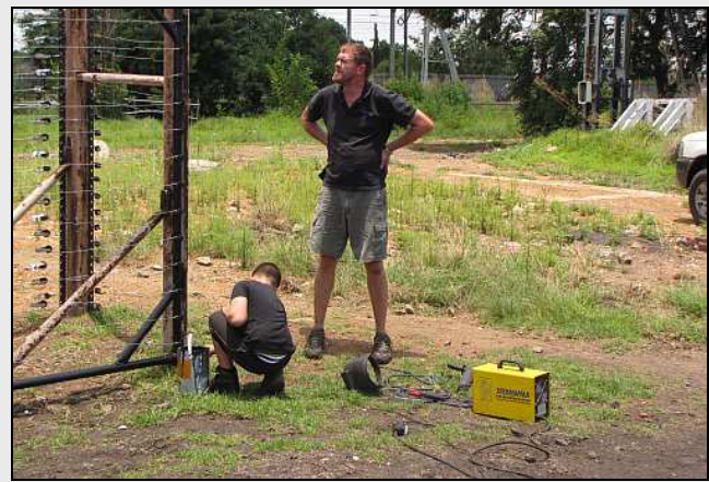
S02 – The Little Man gets put onto painting a recently welded gate stopper, while Long Shanks checks for other signs of rust and missed paint on the previous day's welds. This etching primer dries quite quickly but needs deliberate dabbing on the rougher surfaces and the welding fillets.
