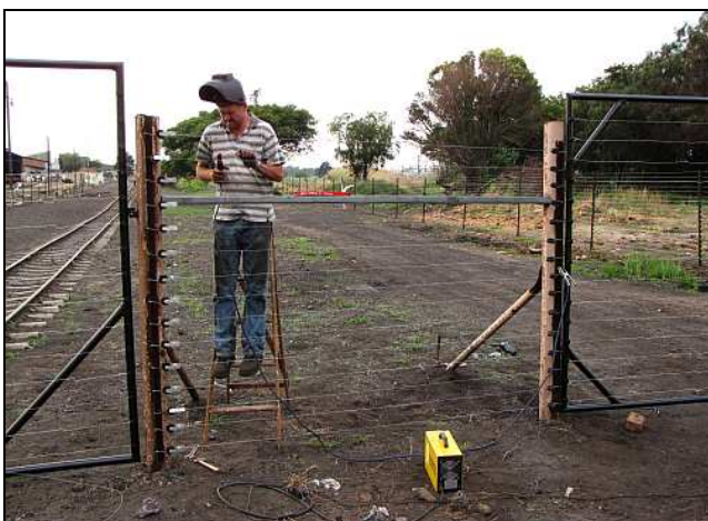
G23 – About an hour later now. (I had been wiring strands, so no photos for a while.) The corner and intermediate panels are strung as well as two of the three gates. Shaun is checking the cooling welds on a spreader bar. Not only do the opposing diagonal braces now assist each other, the latch was in better alignment. (The poles were diverging.)
