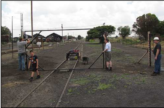
G01 – This is the railway gate that was fabricated the previous week, complete with painting and the insulators mounted. Smudge (L) is marking the gate post for the new hinges. Gabriel Blore is trying to get out of camera range.
