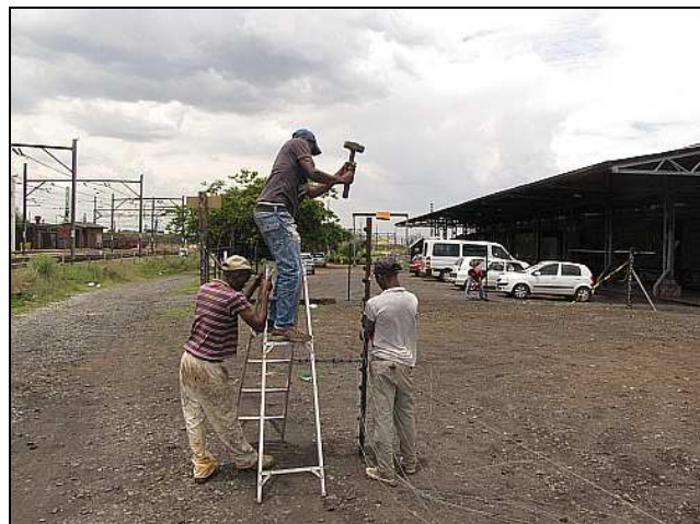
E02 – The existing poles were tapped in (no foundations) for speed. When you have a steam depot with four scrapyards in the vicinity and bracketed by squatter camps, you don't dare leave your perimeter open even overnight.
