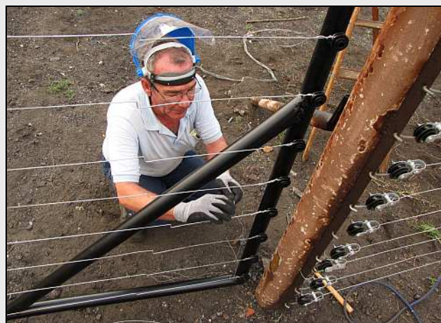
G24 – As soon as the welds were done, Gordon got started on the jumper wires. We wired our western gates as a single panel rather than alternating strands. (To eliminate unreliable bridge jumpers on opposite polarity on a moving gate.) As our system has an earth connection to the neutral, it can still detect a short or leak from the gates.
