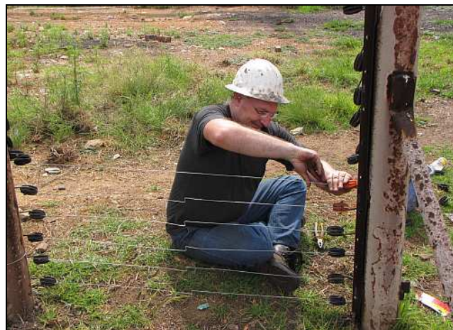
G22 – Once Shaun had finished with the welder and the corner panel clear of sparks and slag, Aidan settles down to trying out installing a few strands. We didn't bother with tensioners or turnbuckles on such a small fence panel – just a few art-deco style zigs and zags to tension the wires.
