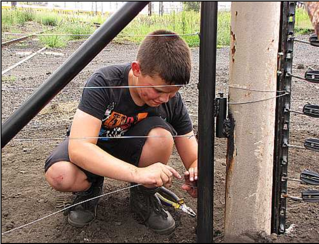
G07 – Gabriel Blore (Stepson of The Smudge) has a go at the other end of that fence strand. He is just discovering how stiffly uncooperative that galvanized mild-steel wire can be, and you go twice around those little bobbins. The Y-Standard bar is welded on – the tie wires now unused.
