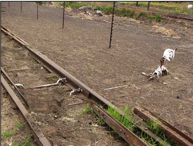
E07 – These long-disused points survived 100% intact, even with the tumbler outside of the original fence. They need to have the point rodding trench dug out and the slide-pads cleaned n' lubed before going back into service.
