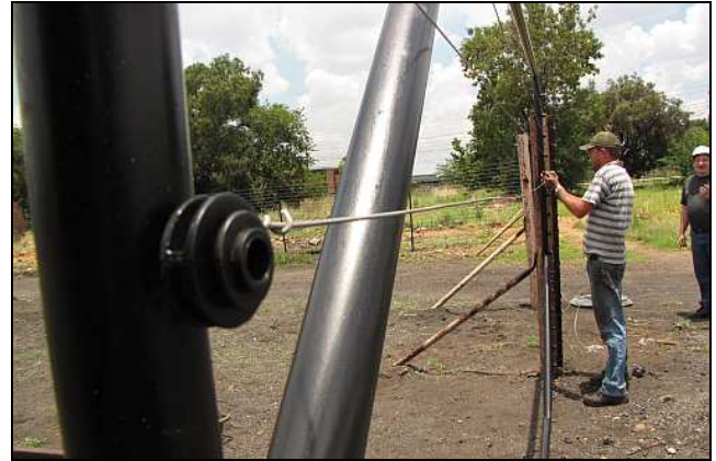
G02 – For economic reasons, all of the new west gates use simple bobbin insulators at both ends. Once the wires have settled in service and re-tensioned via kinking, the chaps will then fasten extra bobbins onto the diagonal braces.
