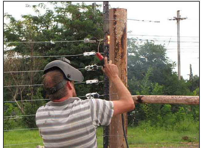
G14 – After tea, it was time to prep the poles for the road vehicle gates. Here, Smudge has just been welding a temporarily tied-on Y-Standard pole. The corner pole is a boiler flue pole that was originally erected by Andre v. Dyk.
