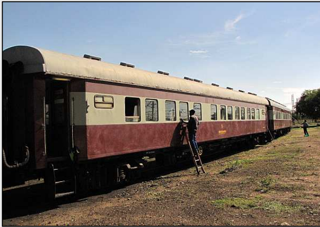
P03 – The entire sleeper coach set was given a circus-elephant style scrub down and all the exterior windows cleaned. There wasn't enough time to redo the cobra wax polishing, however, but it was still quite an improvement.
