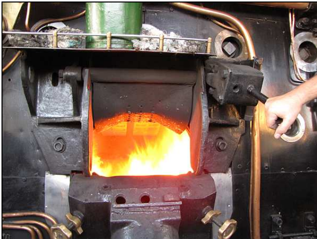
P14 – Reefsteamers fireman, George Hoddinott, took on the challenge of firing this mech. stoked locomotive by hand, and proved it can be done even through that narrow, winged portal. Hand-firing 3046 was one of the inspirations for the present repair work on 'hand bomber' 15F 2014.
