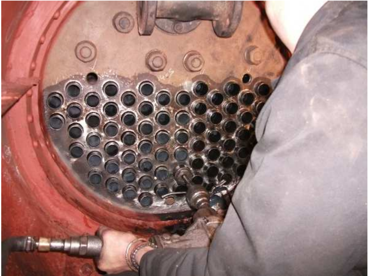
Expanding the smoke box end
