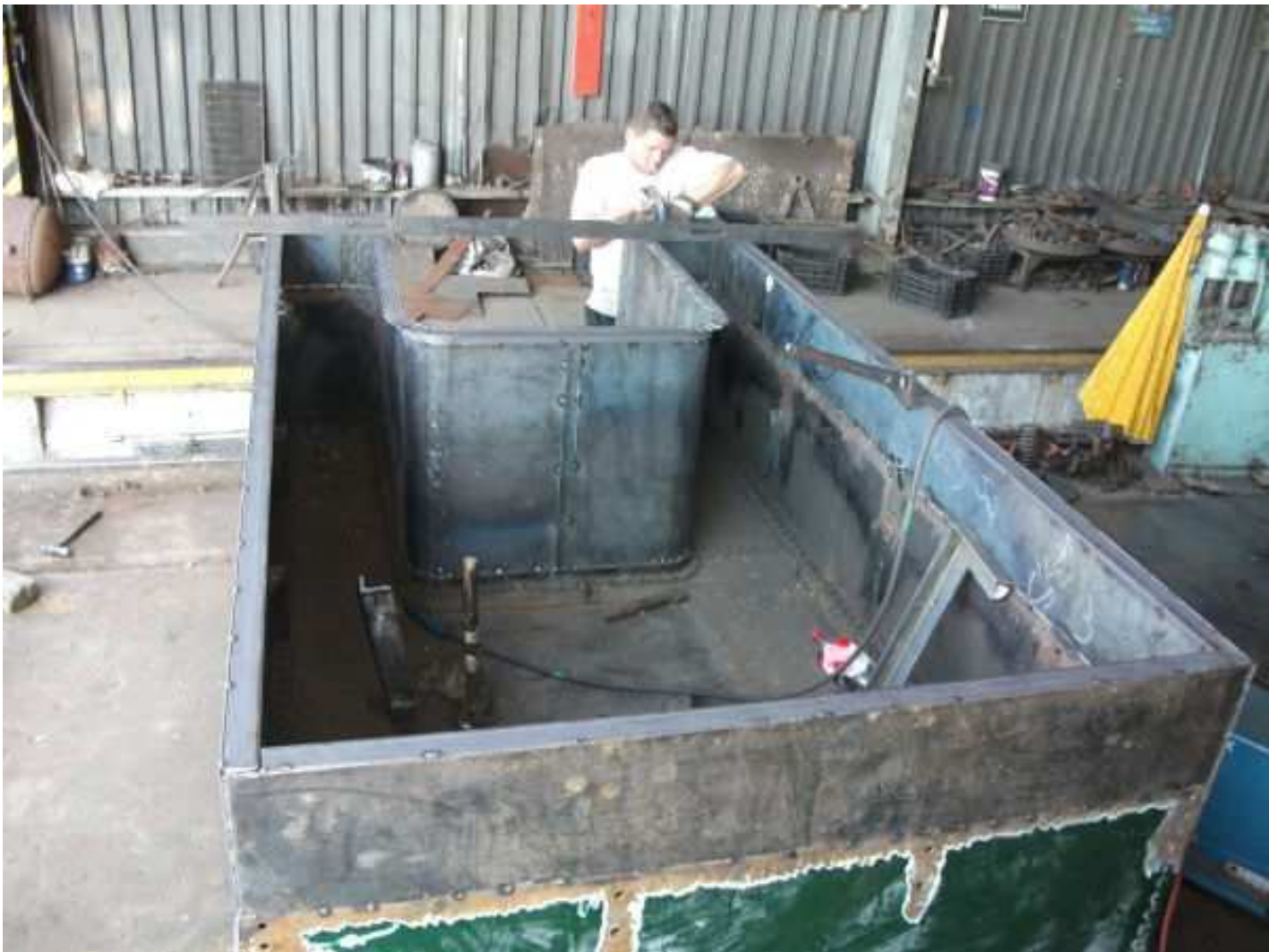
Bottom half of tender renewed. Rivet holes to be drilled and tank to rivet.
