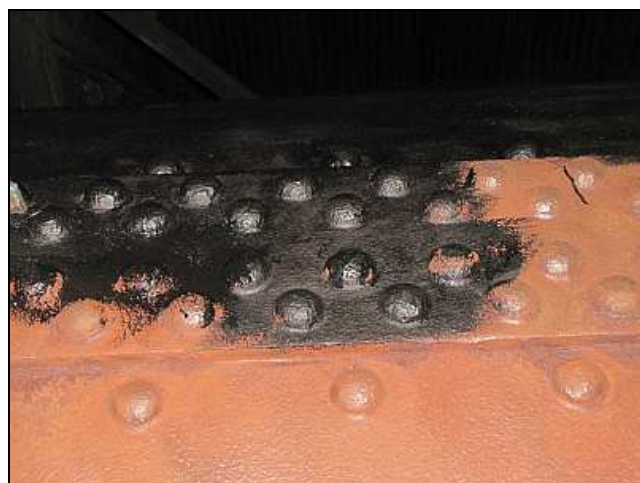
B10 - A closer look at the start of the priming job. Even though the loose rust has gone, the aged surfaces are still a bit pitted. This requires tedious pushing strokes of the paint brush to fill all those vulnerable holes with primer.
