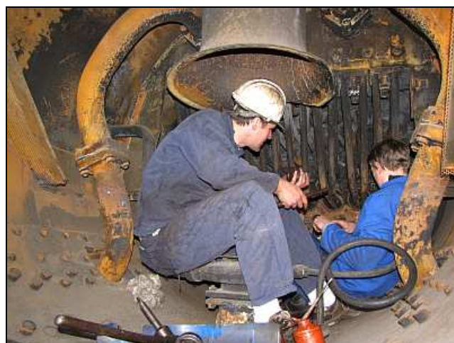
T04 – Swakhart (Left) and Hott-Nutts insert a tube expander to start installing the first of the seven new boiler tubes that they would put in this day.
