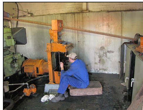
George tackles the lonely job of diagnosing the faulty starter, with neither wiring diagram or colour codes available.
