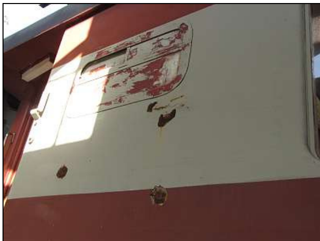
C11 – This rust pattern is unusual. We believe it to be from chemical fumes rising from the toilet (Bleach or Ammonia) from when the coach was standing plinthed and coupled to the Locomotion Restaurant in Weenen. The majority of the rust on our coaches had started from the inner panel sides.
