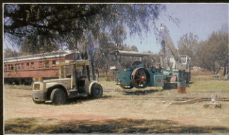
Sandstone's crane and forklift are employed to raise the dead Aveling roller over the railway lines.
