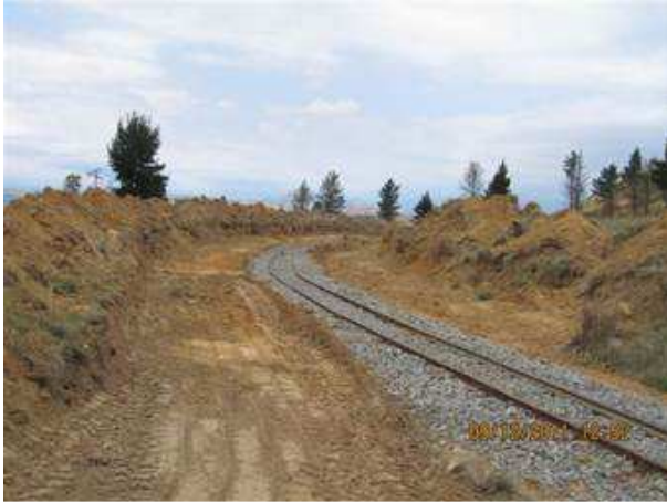
We are reducing the curves at Pandora and putting in additional drainage.
