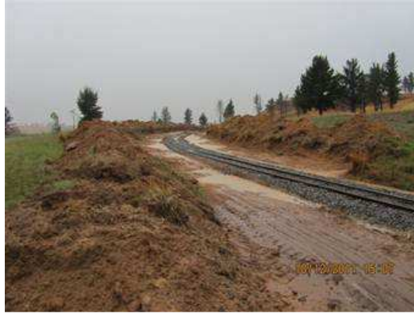
We are reducing the curves at Pandora and putting in additional drainage.
