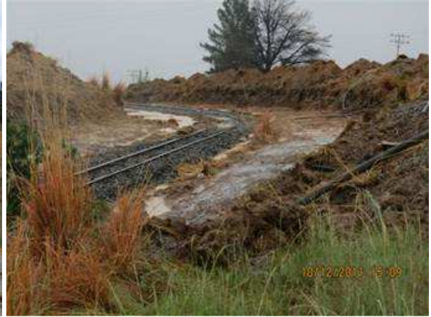
We are reducing the curves at Pandora and putting in additional drainage.
