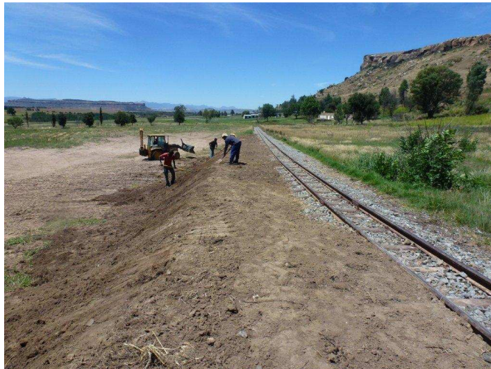
The embankment has been widened and strengthened.
