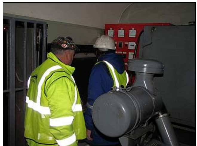
P20 – Training the Train Manager. Dennis Edgar gets a run-down and (simple) start-up procedures presented by Alan Lawton. The gen-set has a strange, almost-spooling startup from cold, but fires up within less than 2 seconds.
