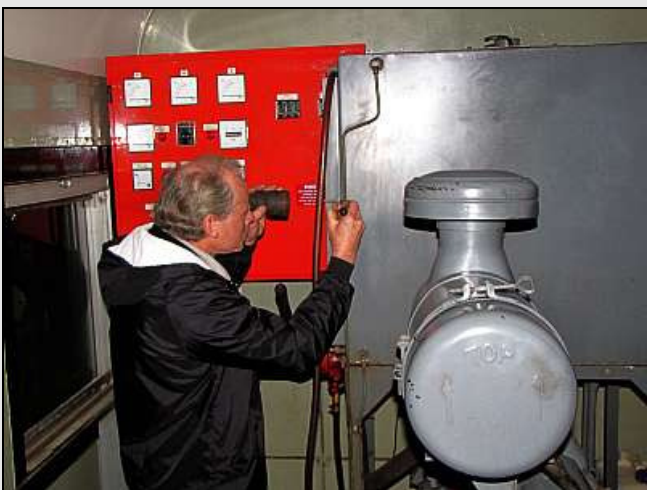
P19 – Engineering Mngr. Andrew King went along for the gen-set's first ride although it had already run for 9 hours while powering the coaches. Here, Andrew is marking the fuel level in the gauge glass to check fuel consumption.
