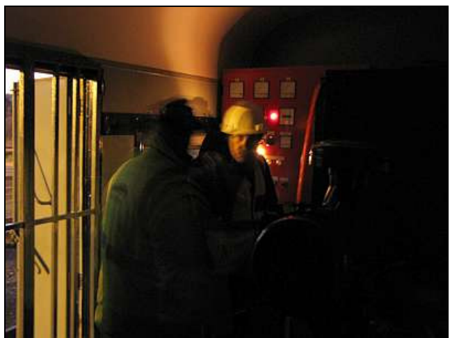
P21 – The white lamp sez that the 12V starting battery is under charge. The red light indicates that the generator's stator is live. The load hasn't been switched in yet, so the lights are still dark and the 3 ammeters all read 'zero.'
