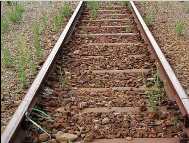
P41 – The outer loops and sidings at Ficksburg are still iron-pan sleepers and 4-bolt fishplate joints, except for the newly laid bypass track in the grain yard. Noteworthy here is that the fishplates have all eight bolts intact and tight.
