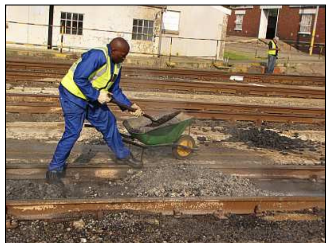
P28 – The Bethlehem service areas are drain shafts and not proper ash pits, so the ash has to go elsewhere. These days, you simply don't dare leave ash on Transnet lines – but it makes sense as it gets sucked into traction motors.
