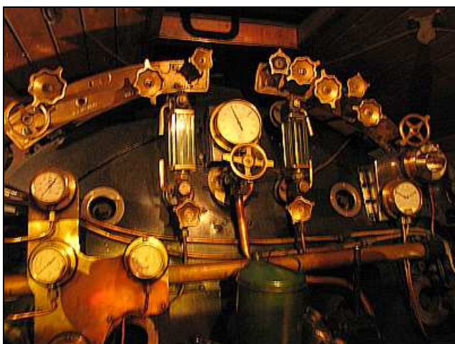
P21 –The rotten sods who took the last leg as pilot crew left the pressure midding, but didn't top up the water. So I had to fill the boiler AND stabilize it on my long overnight shift, with the consequent hit in the coal consumption. Grrr!
