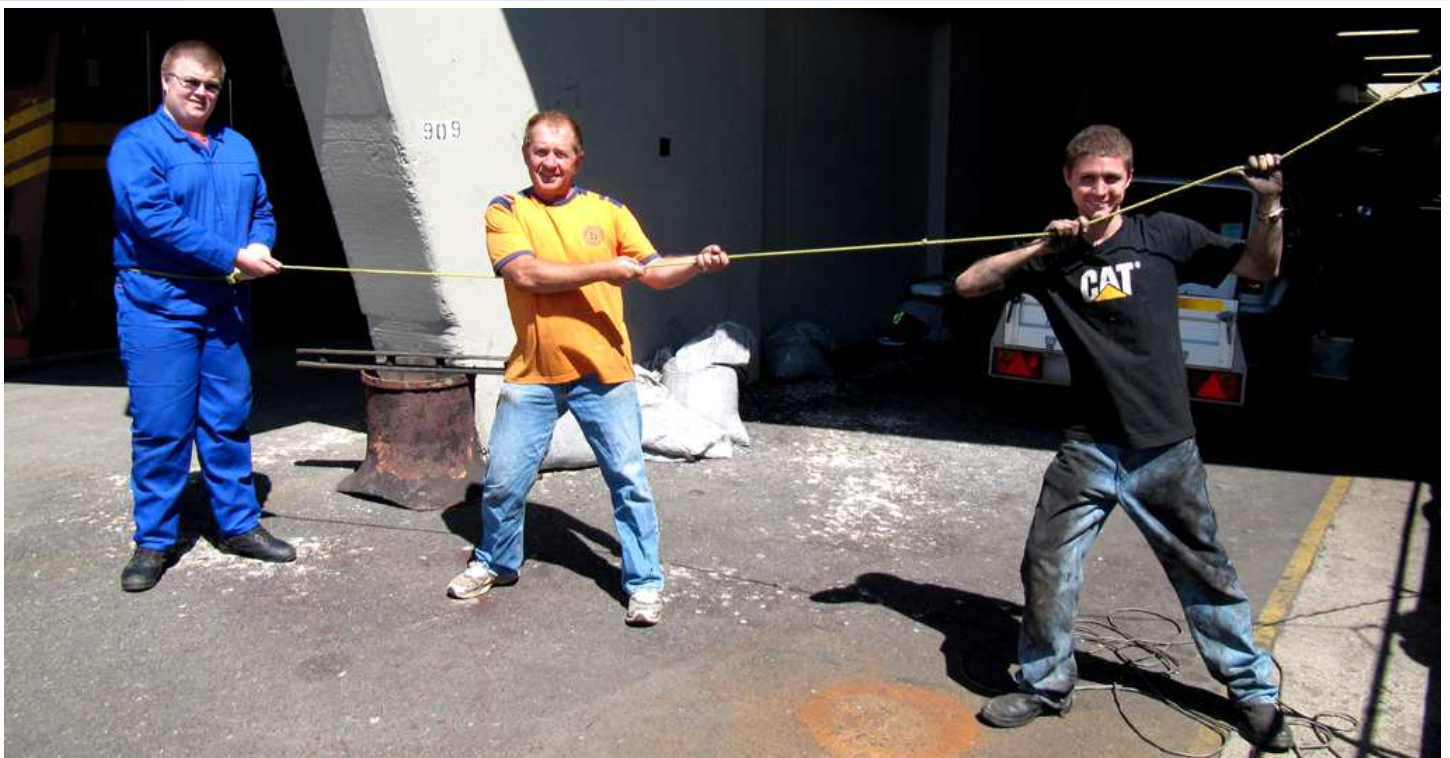
Muscle Power! A lot of tractive effort was needed to raise the new petticoat into position. Photo: Luca Lategan
