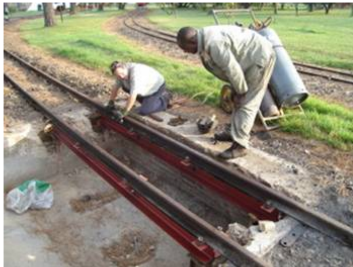
Henk and Petrus securing the rails on the beams, now only needs the concrete blocks around the upright beams.
