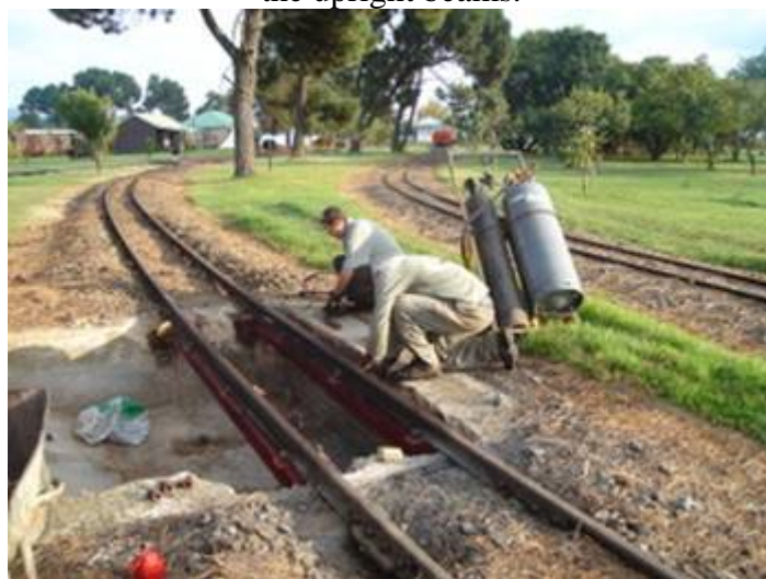
Henk and Petrus securing the rails on the beams, now only needs the concrete blocks around the upright beams.
