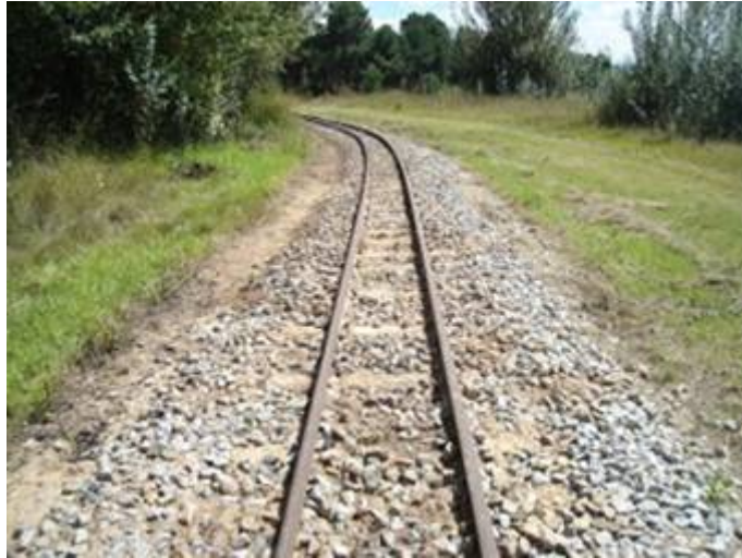
A much better aligned curve near the horse shoe curve between Vailima and Vailima Halt.
