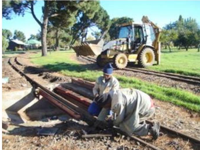
The rails being fitted back with the new beams in place.
