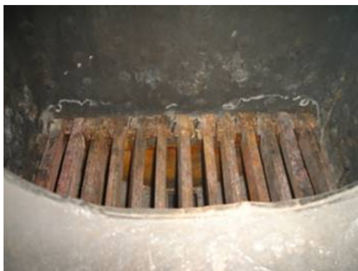
The much wider gap between the fire bars after Derrick worked on it.
