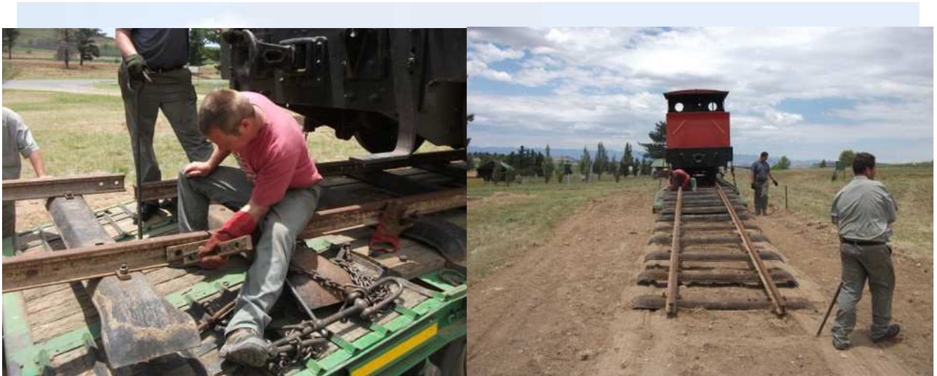
While Henk connected the second panel the rest started to support the ramp rail with wooden sleepers.
