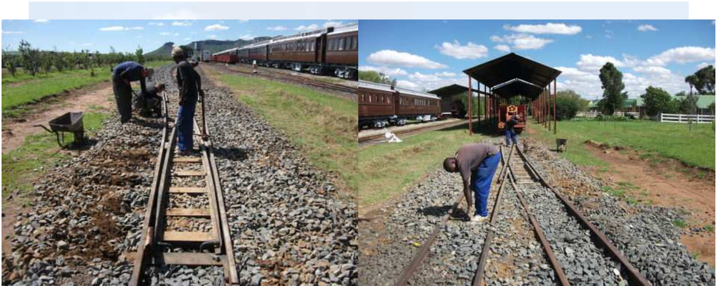
Below: Level ling the first 60 meter of track in the new Hoekfontein Shunting yard.
