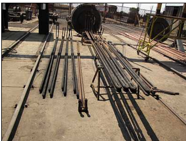
B11 – Pulled Superheaters.
