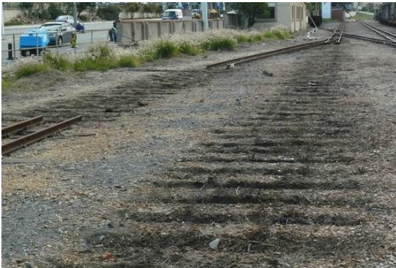
Tracks have also been lifted. It is not known what has happened to all the freight wagons that were parked on these sidings. Presumably carried away as scrap metal.
