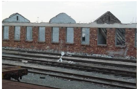
The beginning of the end, of the carpenter's workshop.
