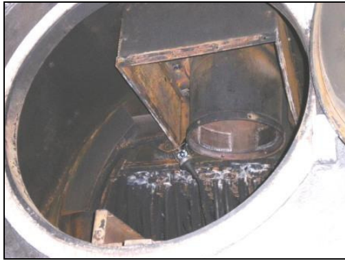
3472 Chimney in place
