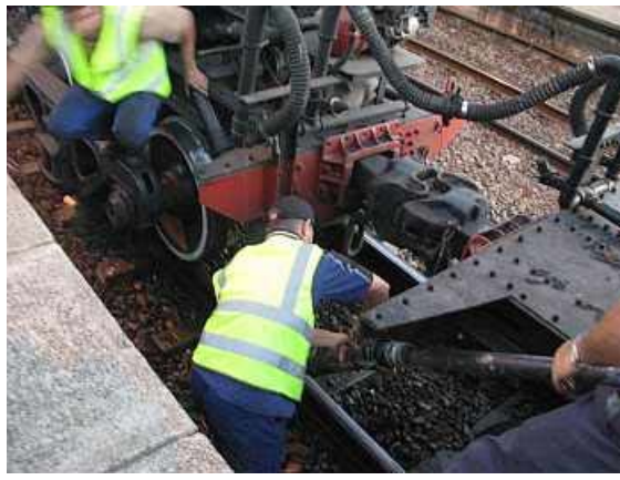
FP52 - Some attempts at line side water line diagnosis after the injectors were starving for water. The front tank car was empty and the rear one still had water. There was a blockage in the common water feed pipe, so it couldn't be bypassed by switching a pipe to the opposite side's water outlet and opening the valves. We got home using the "ballast water" in the front unit's water tank. (The blockage in the rarely used tank car was a build up rust and sludge ) (LG)
