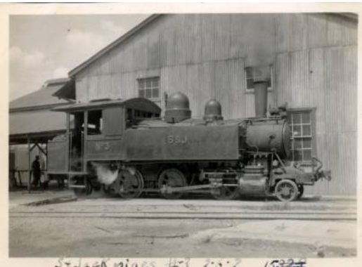
The Porter 2-6-2T in original condition
