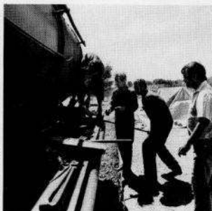
Locomotive work has consisted of maintaining 454 in good operating condition. During mid-1984 she received a complete set of valve gear motion bushes, and overhaul of slide valve components (above). GDA No. 2295 has proved a difficult task for restoration, since after members disassembled and 'cooked' the boiler (above left) a hydraulic test revealed a defective internal main steam pipe which has necessitated the complete removal of superheater elements and header. Hopefully she will be steamed early in 1985, thus becoming the first restored Garratt in South Africa.
