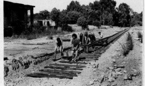
When track work began at the old 3 North Shaft, the present Preservation Centre, early in 1983 only remnants of the former railway lines existed, largely buried under boulders and earth. Just a short portion of the original roadbed was usable and rails were laid on the wooden sleepers (above). A front-end loader and grader were brought in to clear and level the area (above right), after which Preservation Group members learned trackwork the hard way (right), right people to a team.
